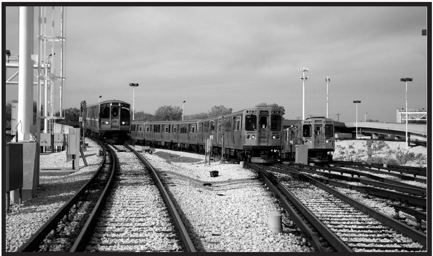
The Howard station at Howard Street and Hermitage Avenue serves as an important transfer point in the Chicago Transit Authority's rail system. The station is served by the Purple, Red and Yellow rail lines pictured here. (From the collection of Bruce G. Moffat)
