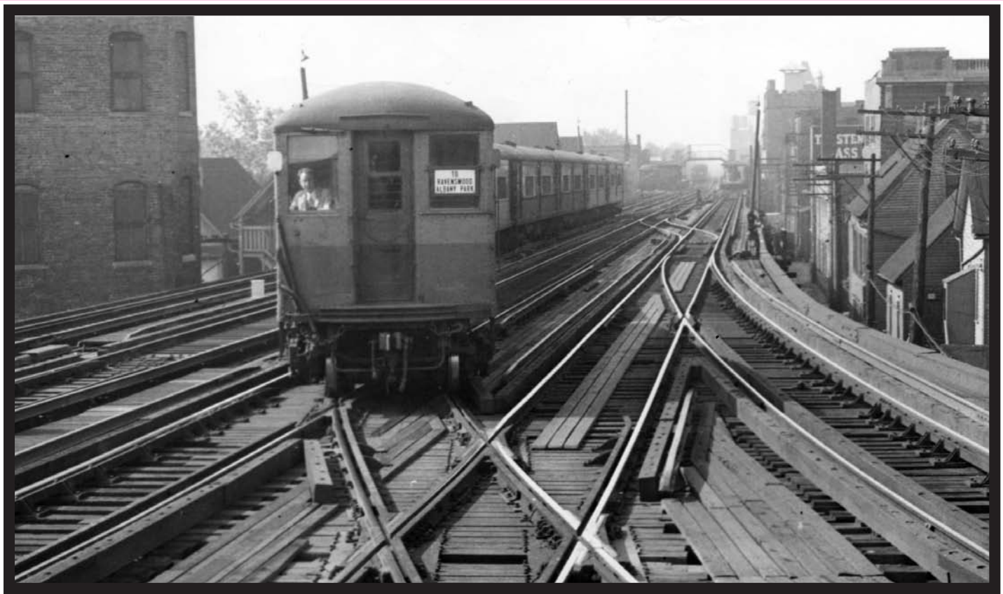
A six-car all-steel Ravenswood train of the Chicago Rapid Transit Company (a CTA predecessor) leaves the 4-track North Side Division main line at the Clark Street interlocking tower. The overhead bridge at the Belmont station is in the background.
