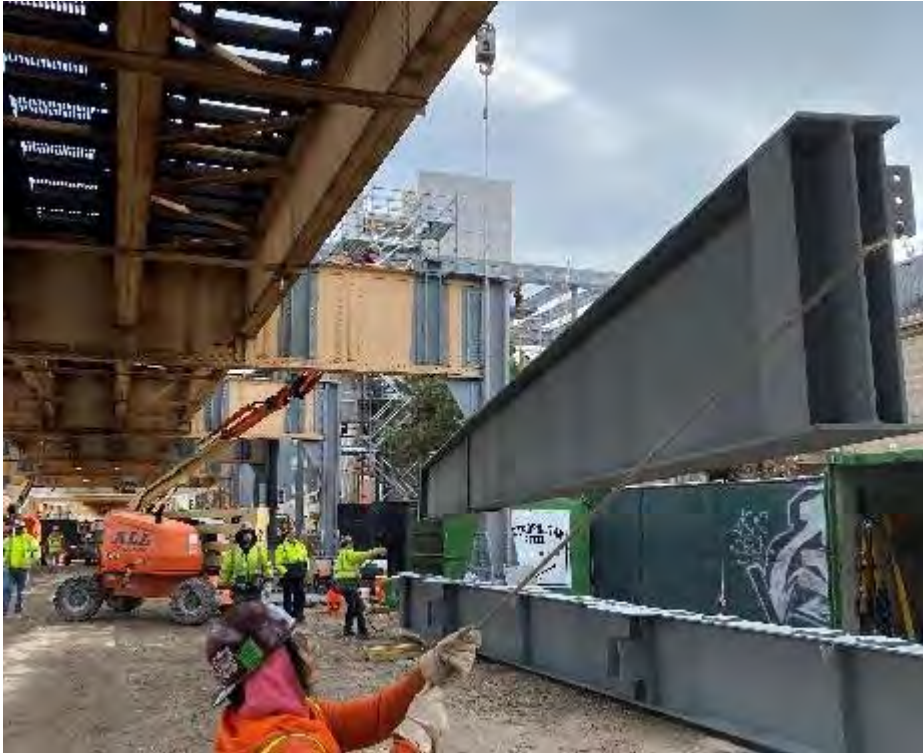
Lifting Platform Steel – West of Station
