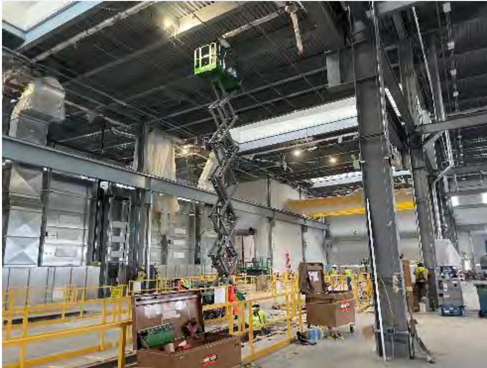
Overhead Pipe Installation
