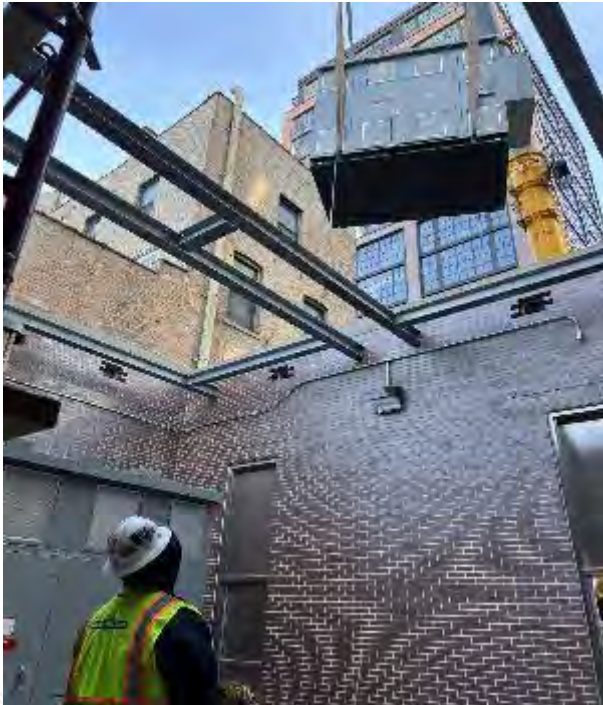
Transformer #2 Delivery and Installation at Haymarket
