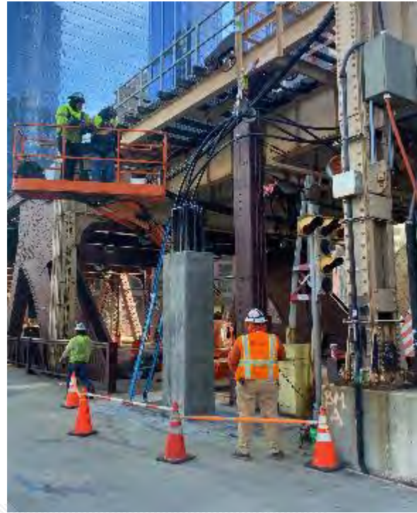
Cable Installation at Canal
