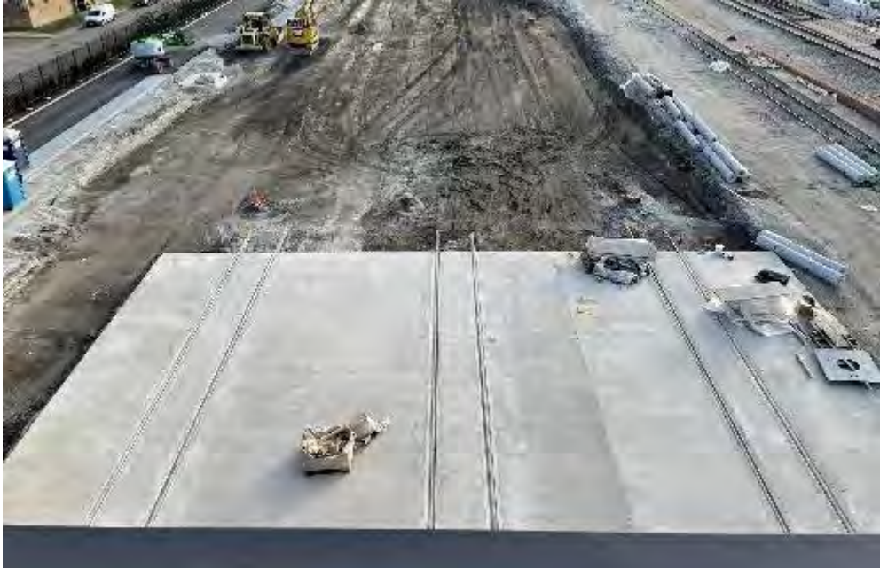
South Yard – Excavation
