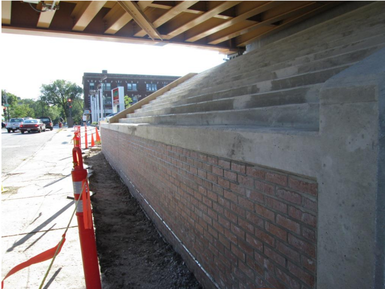
Greenleaf South Abutment – Completed Knee and Slope Wall
