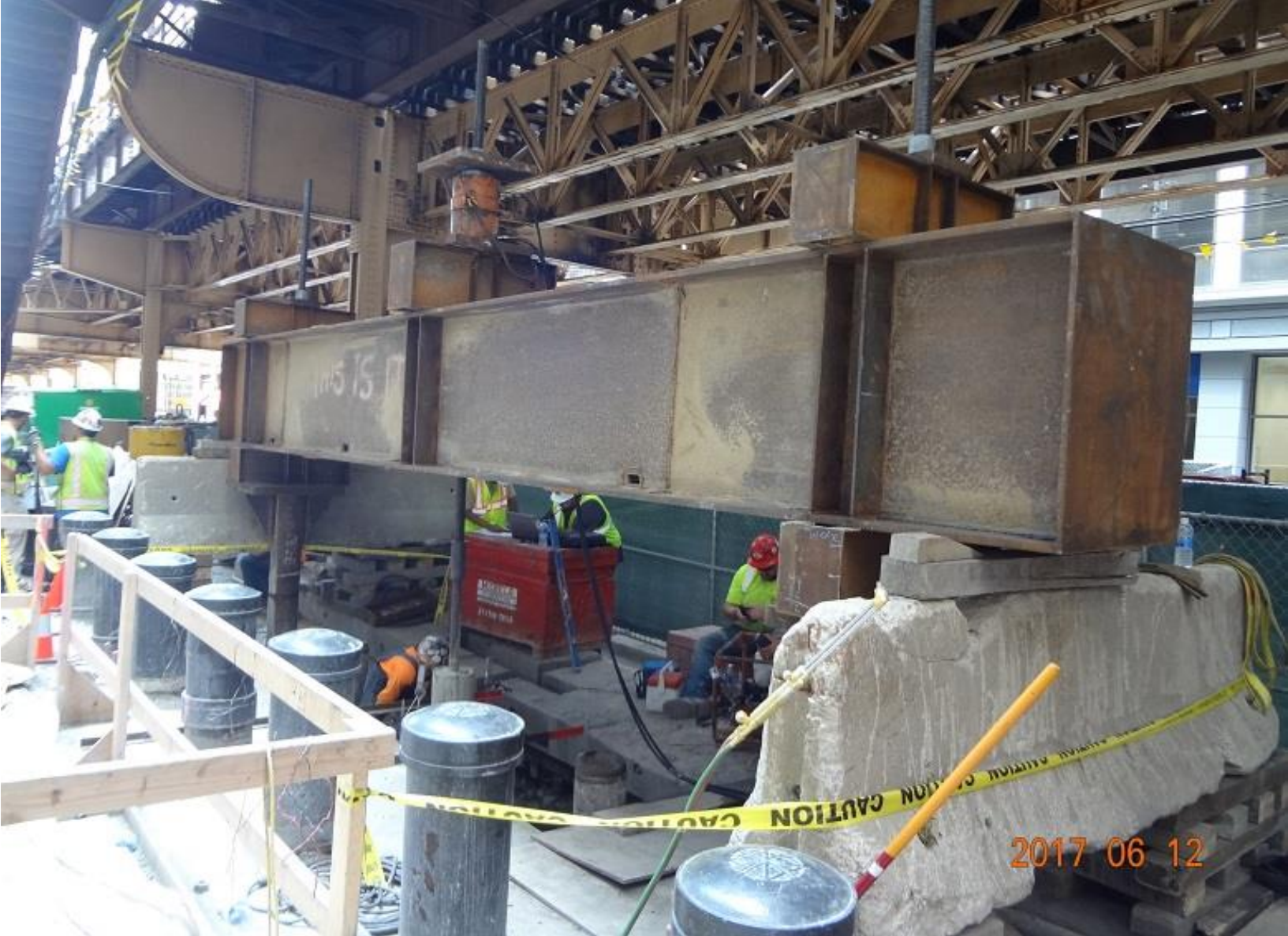
East side - Earth Retention System (ERS) micropile load testing operation
