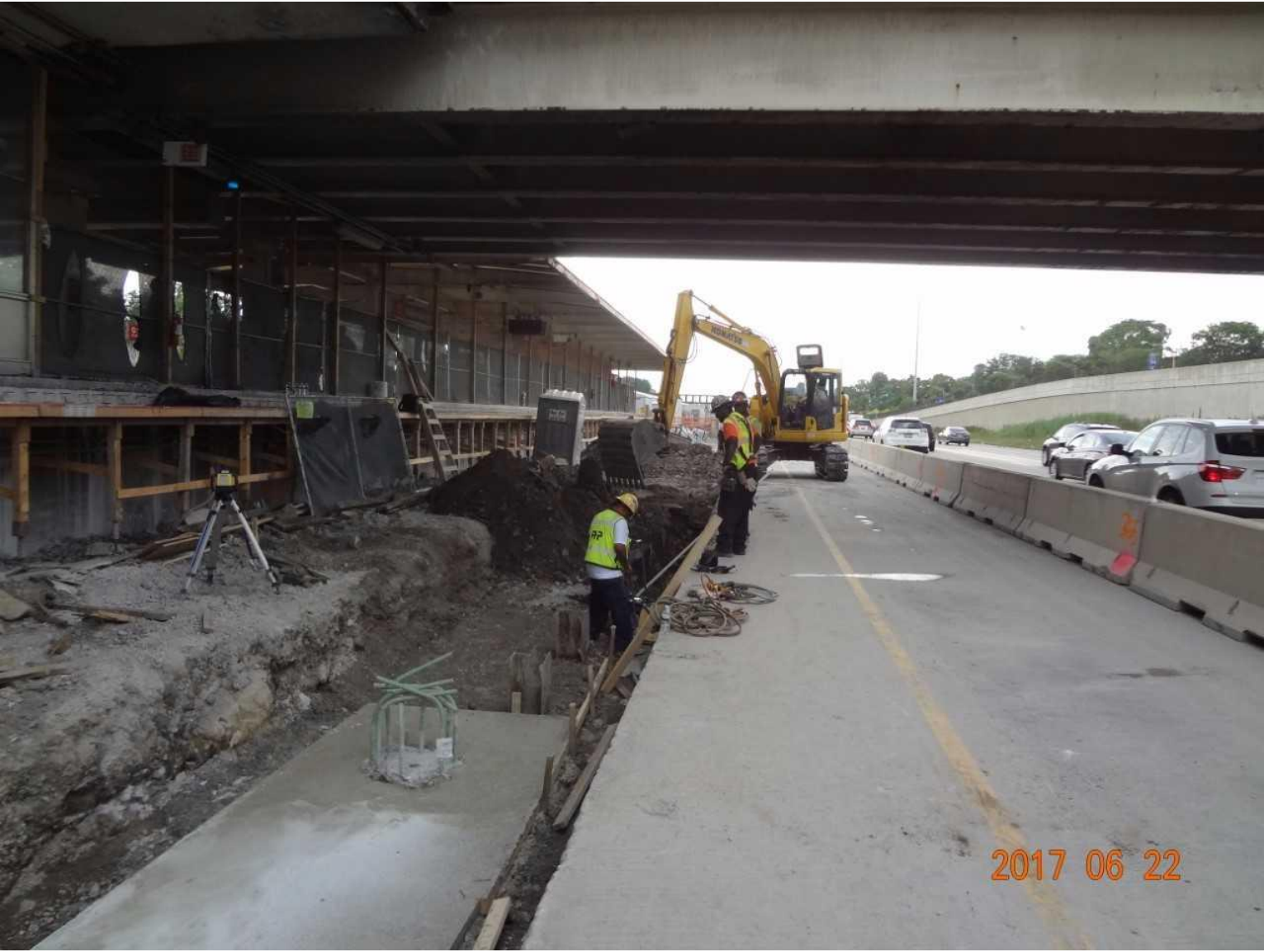
North Terminal foundation and shoulder work
