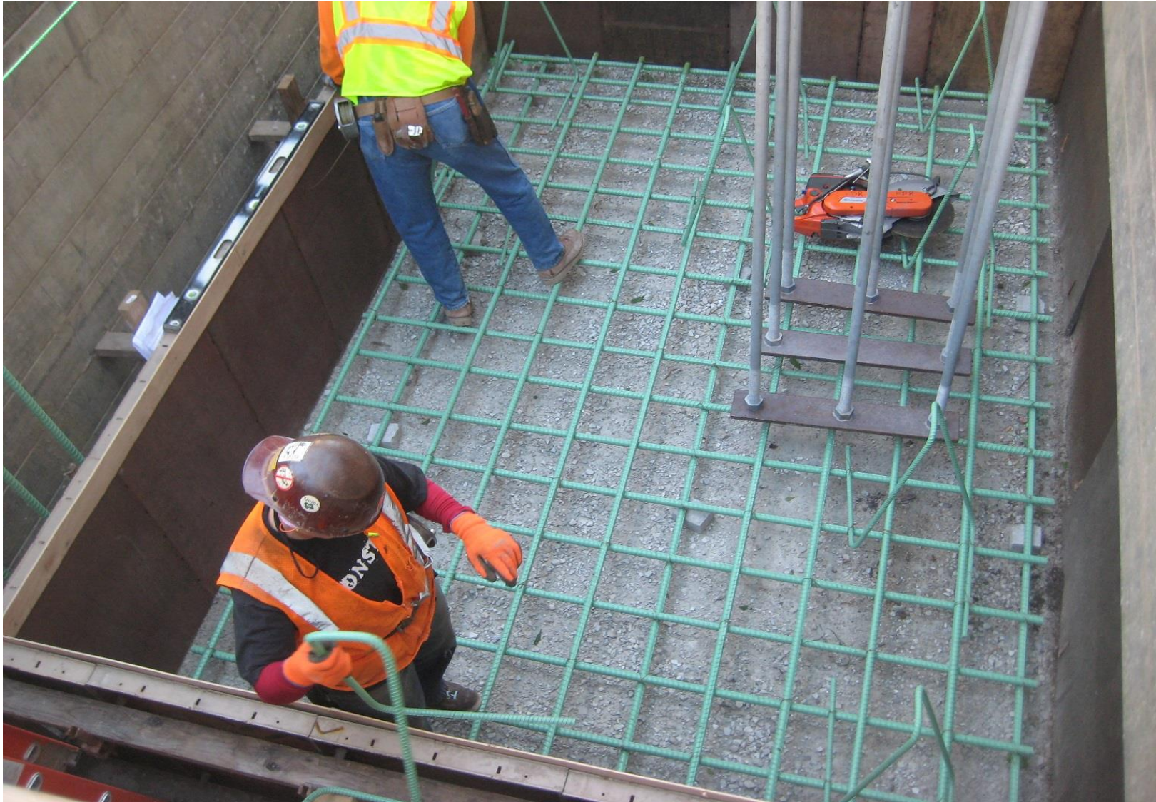
Foundation steel installation at Willow Relay House site
