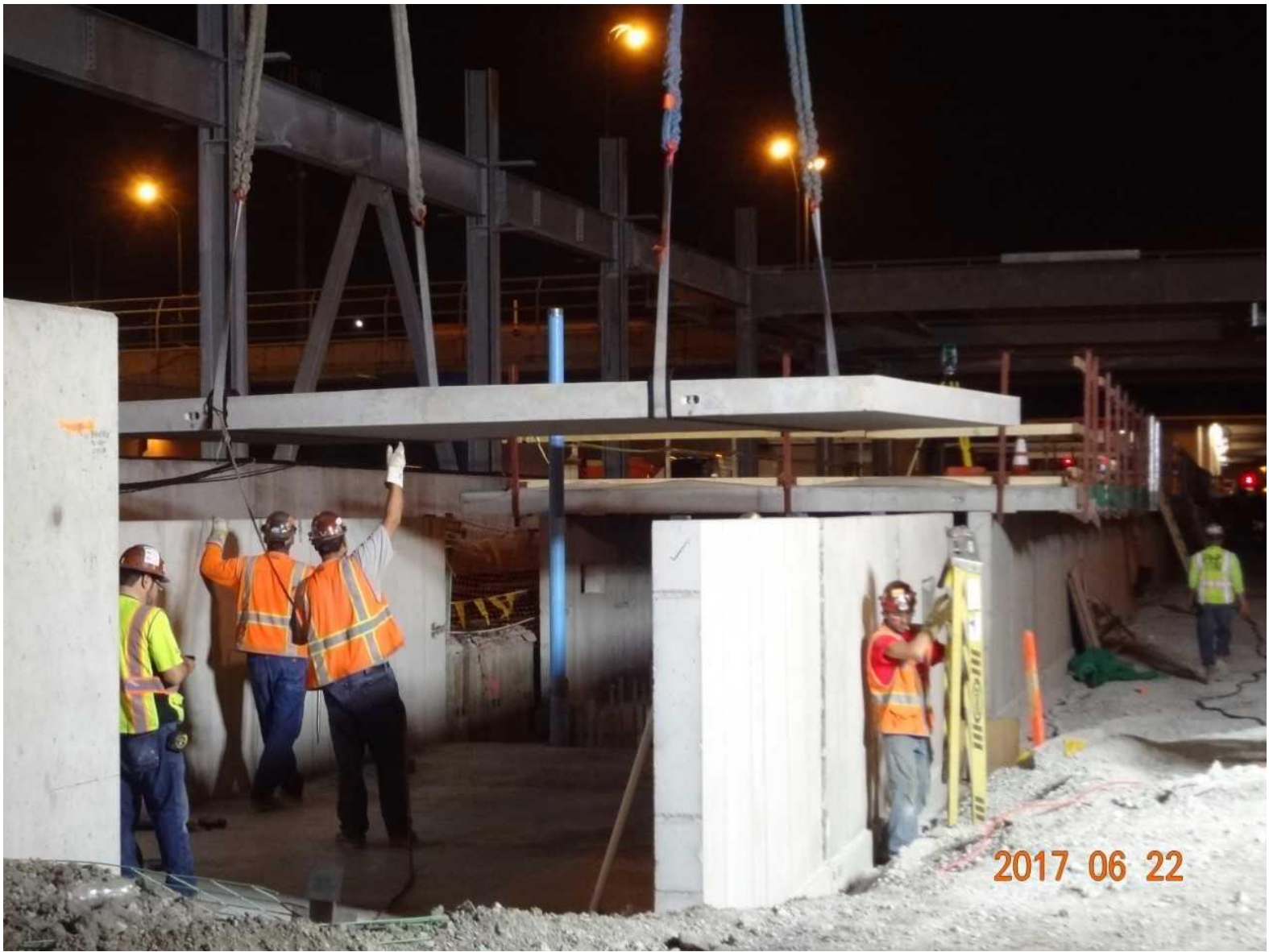
South Terminal platform installation
