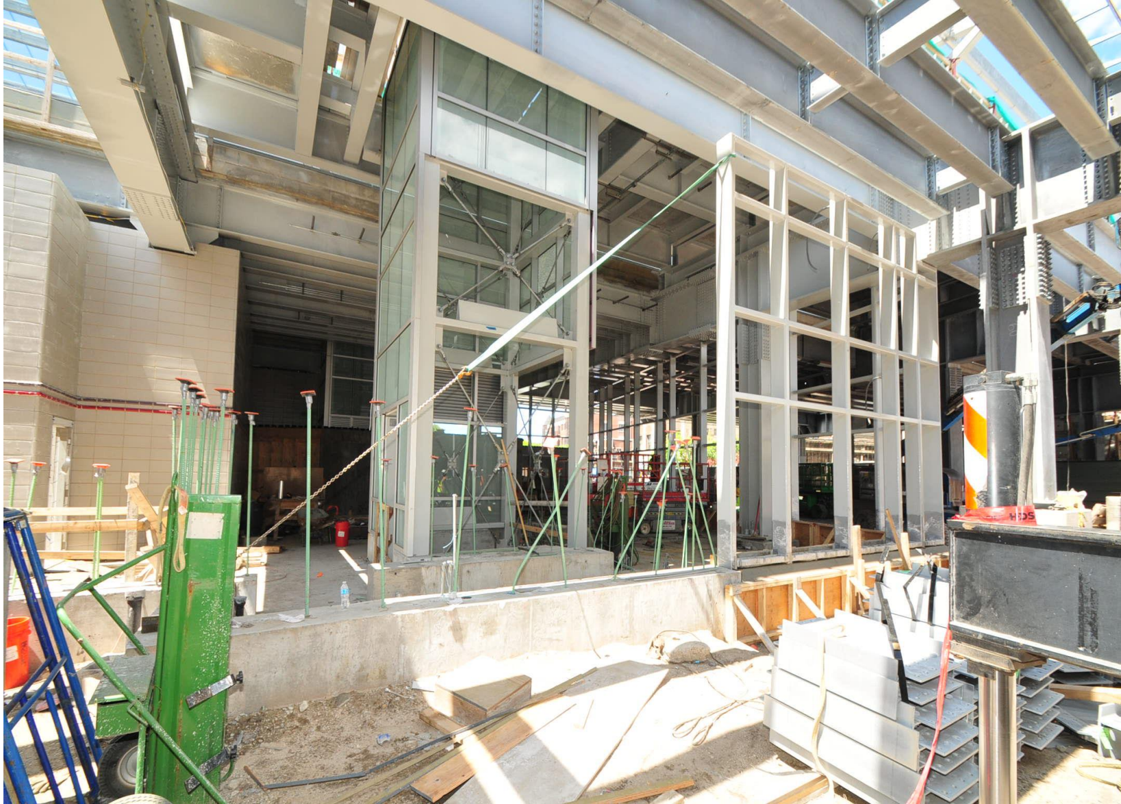
Wilson main station build out
