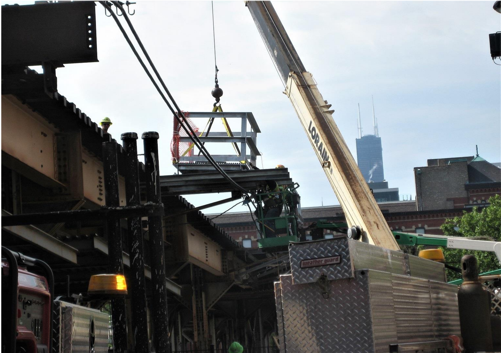
Wayside platform installation
