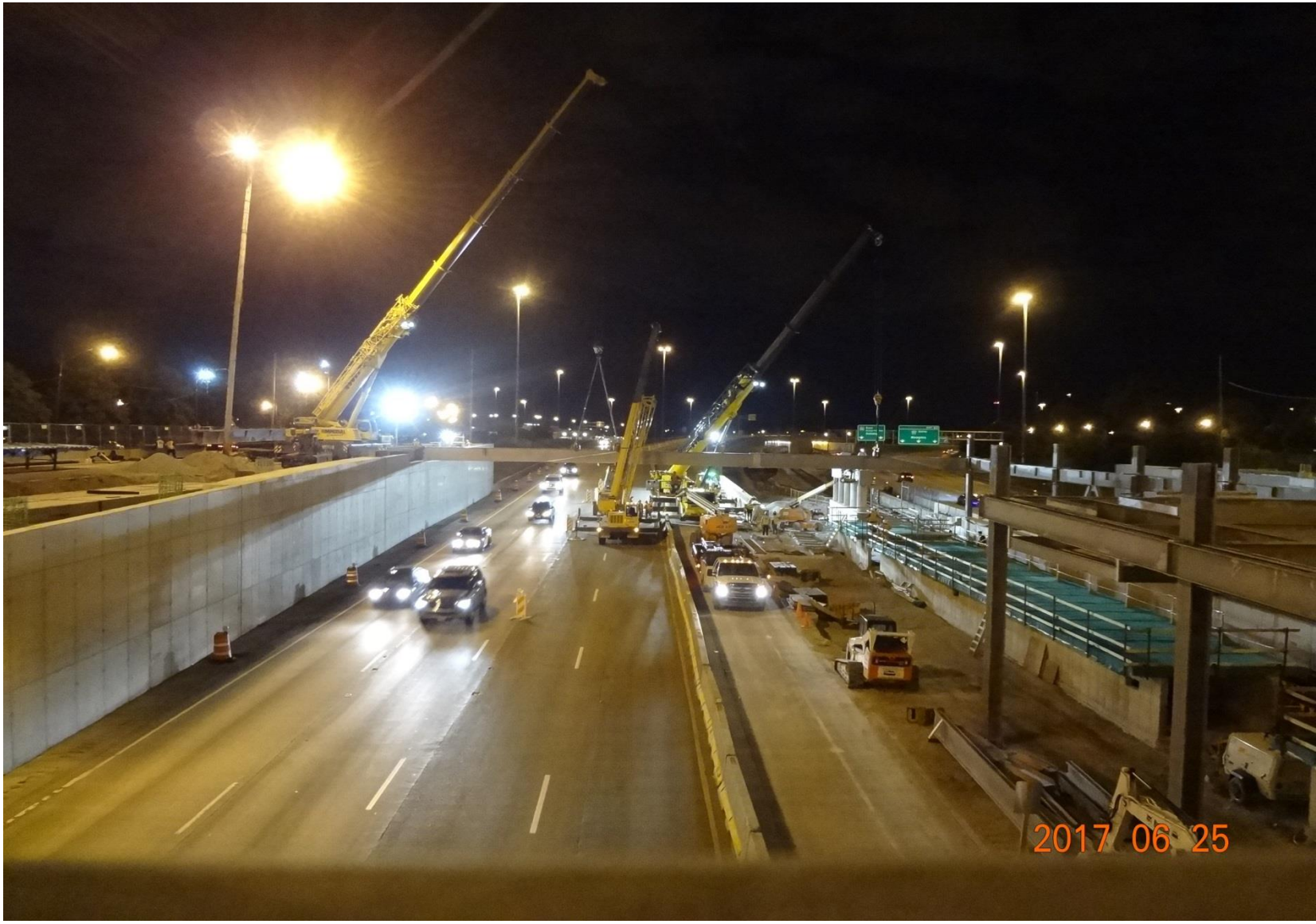
South bus bridge steel installation
