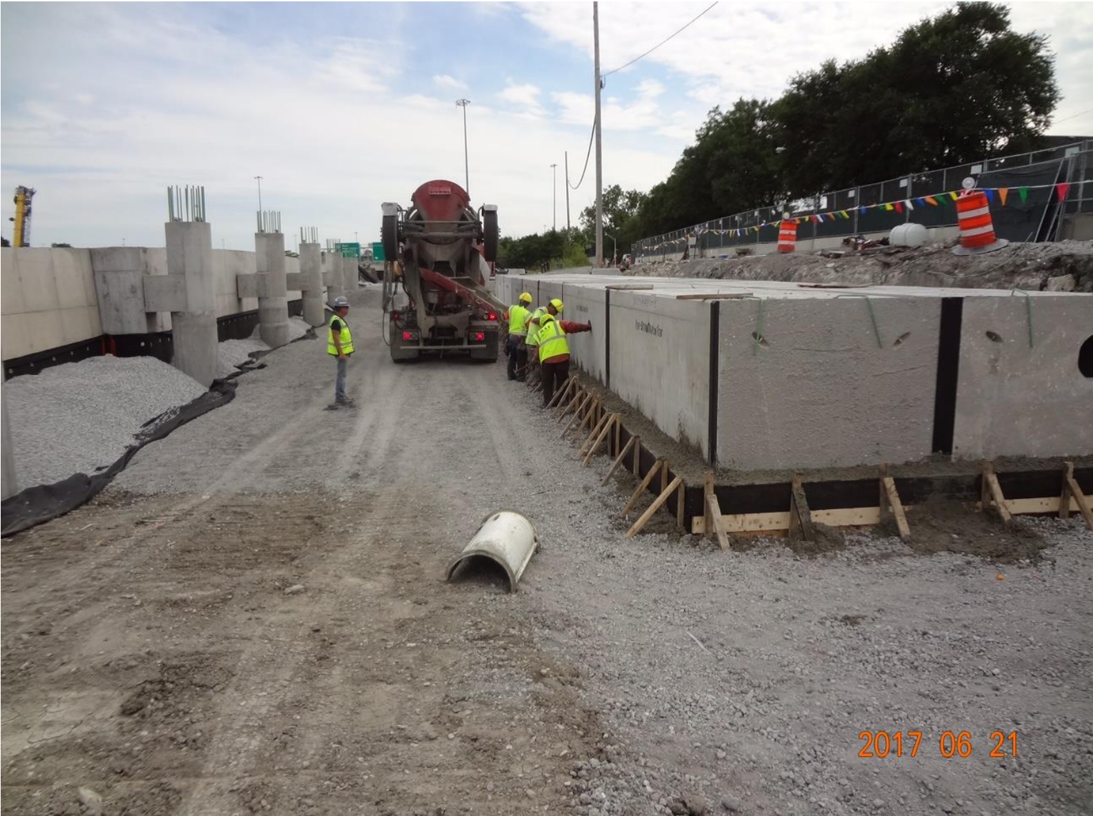
Detention chamber installed under southwest bus turnaround area
