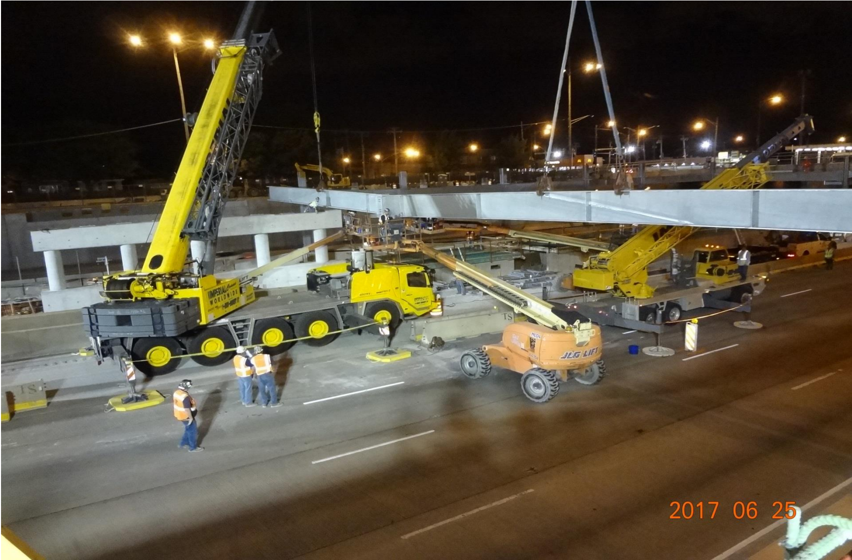
South bus bridge steel installation
