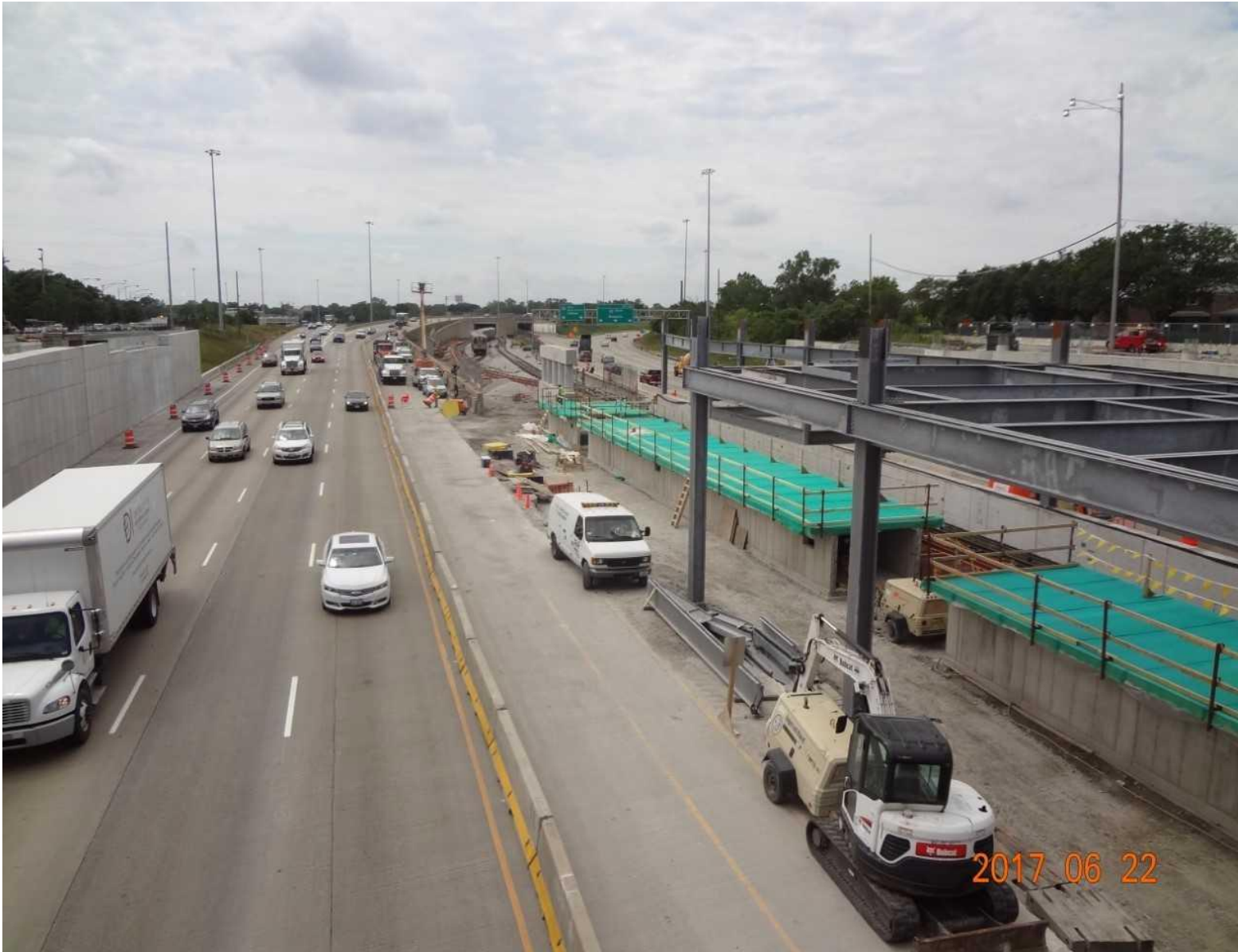
South Terminal building steel and platform installed
