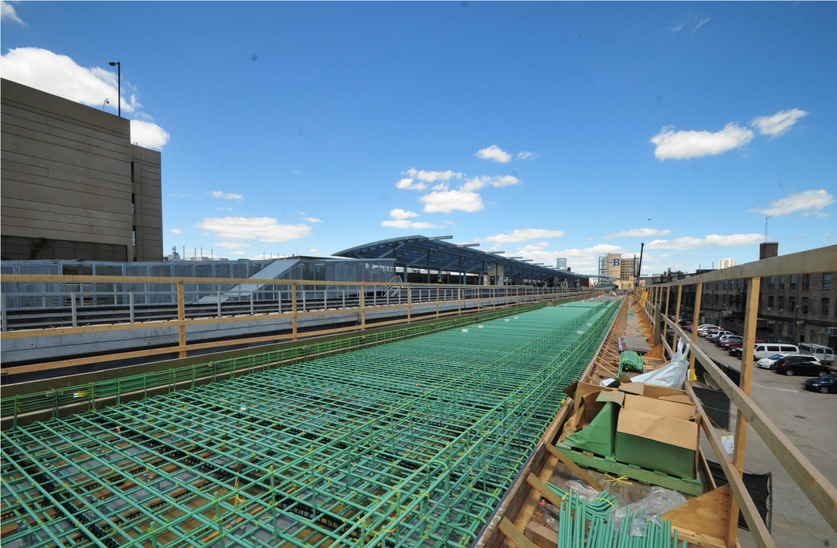
New track 4 rebar installation
