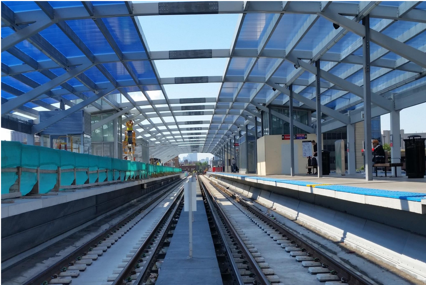
New east platform and canopy steel structure
