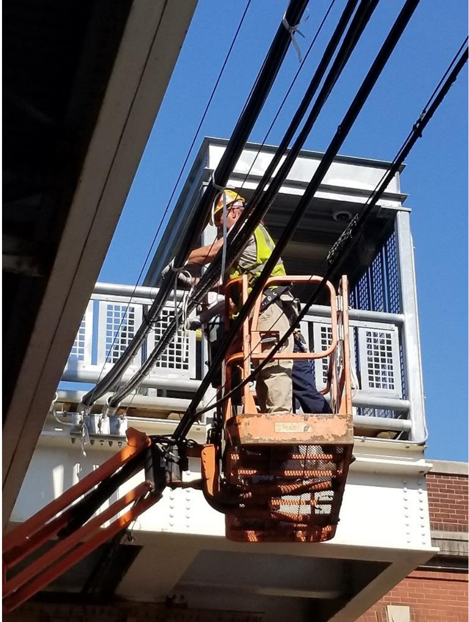
Pulling and tying of signal cables
