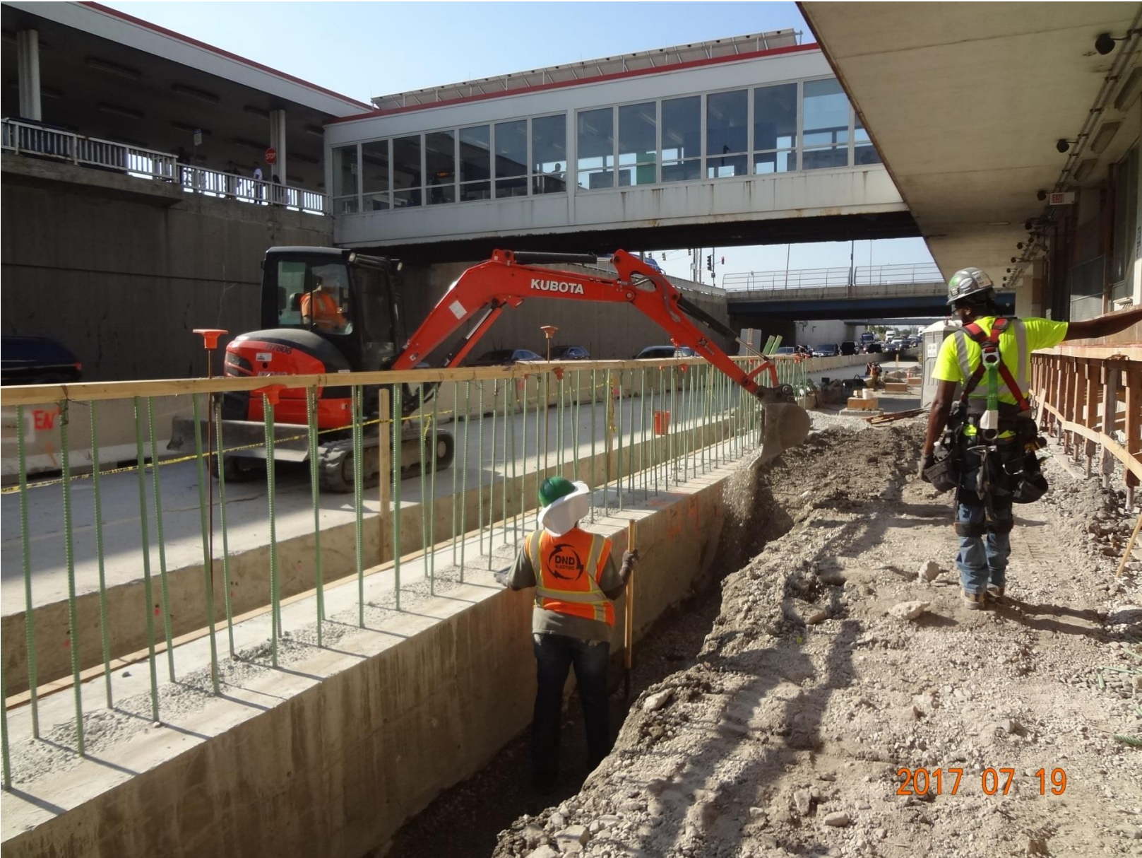
North Terminal East Side Foundation Installation
