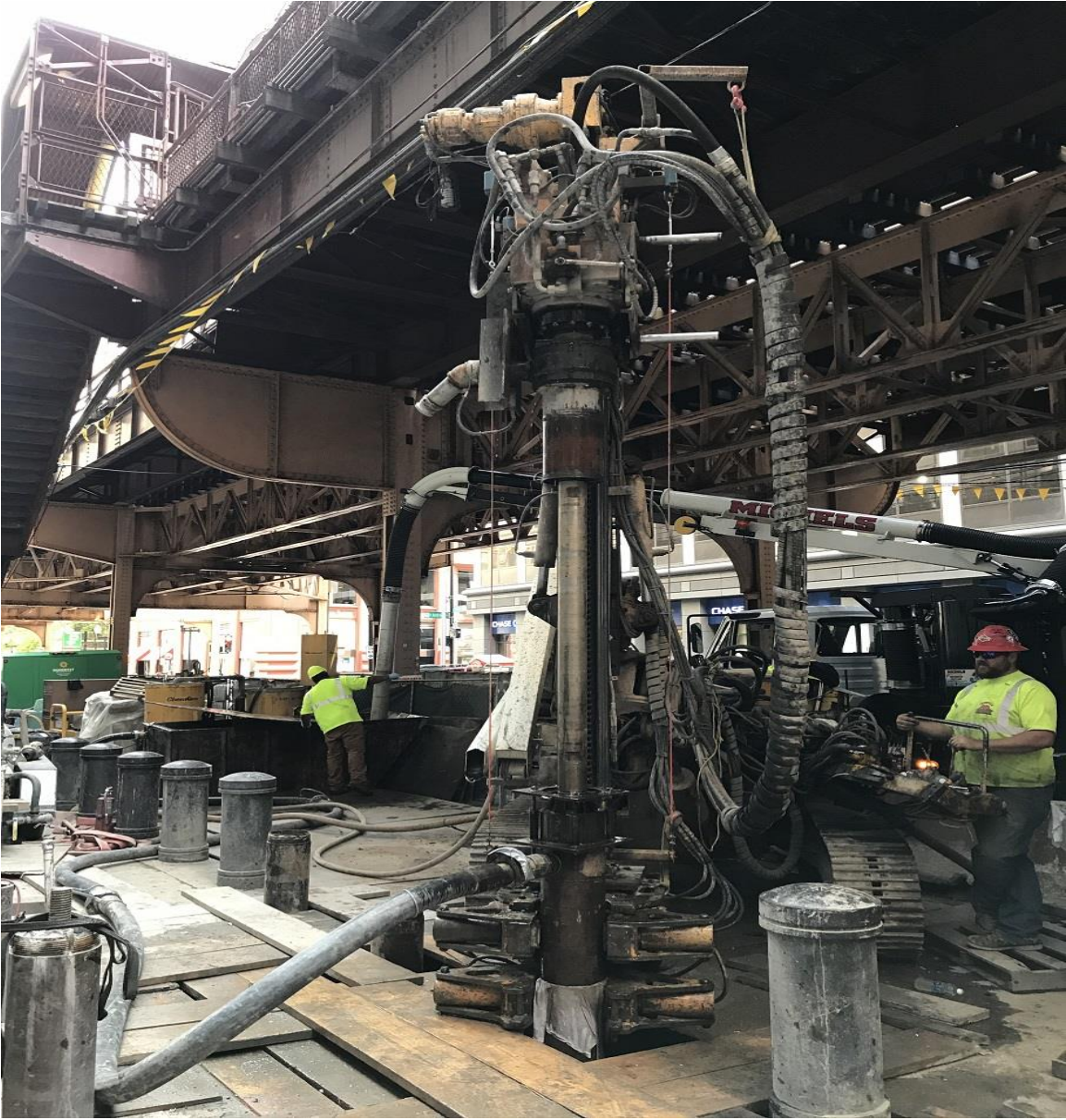
East side – elevator micropiles
