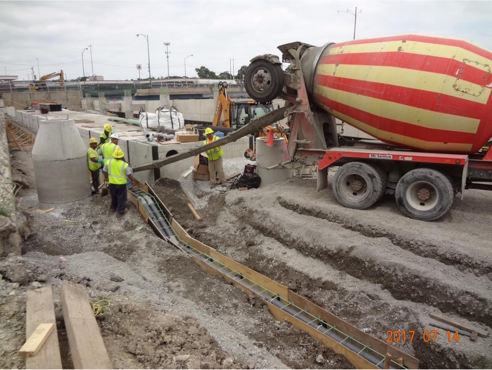
Electrical Ductbank Installation under west side Bus Turnaround Area
