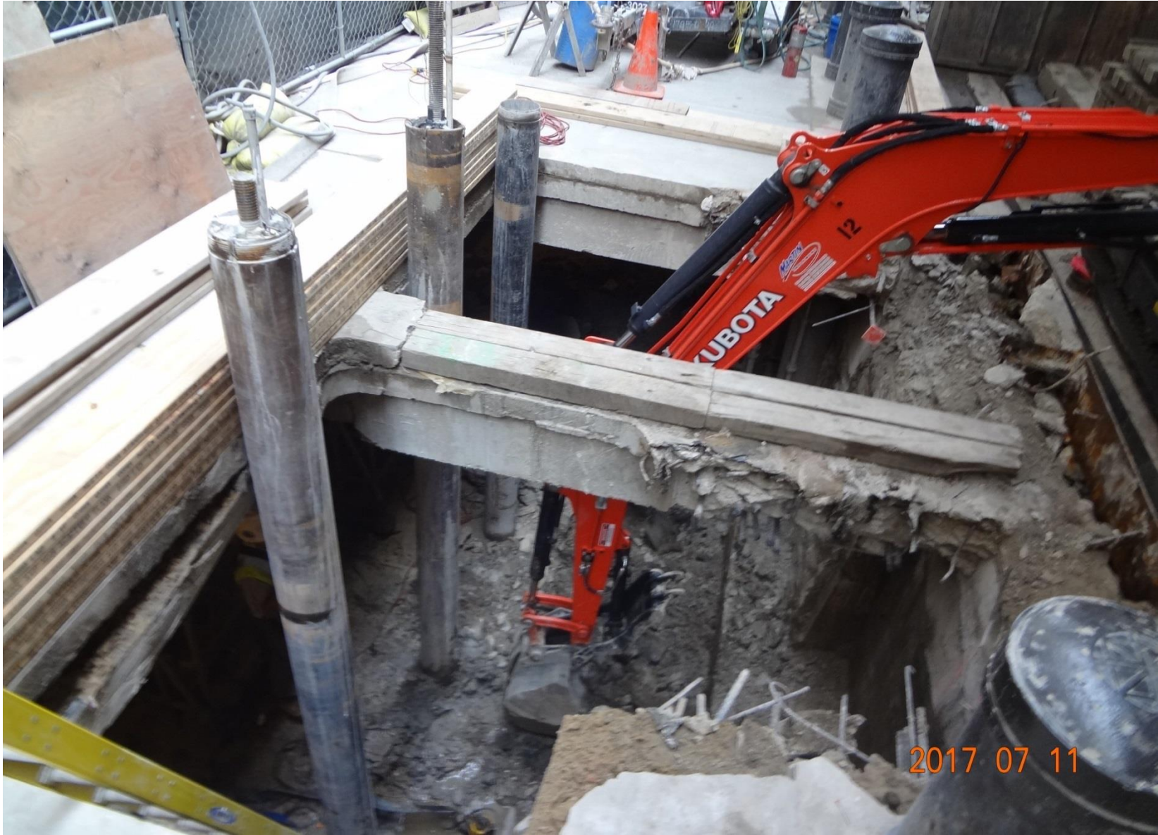
East side – demolition excavation for elevator micropiles
