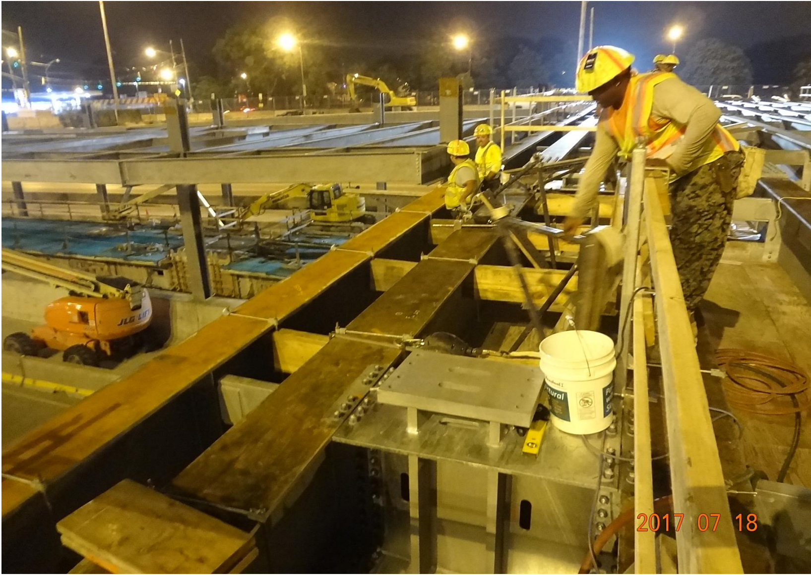
South Bus Bridge Steel Detailing Work
