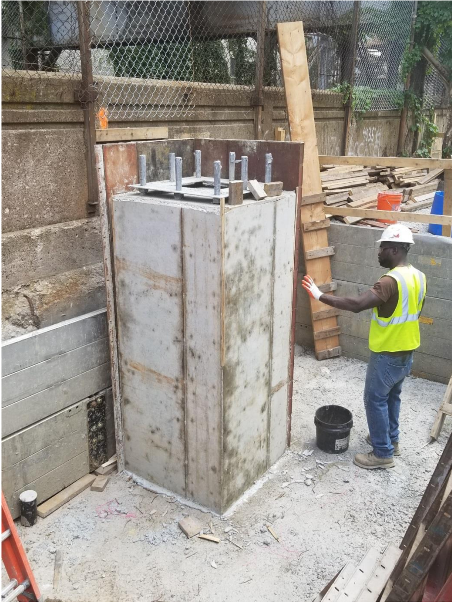
Form removal for Willow Relay House foundations
