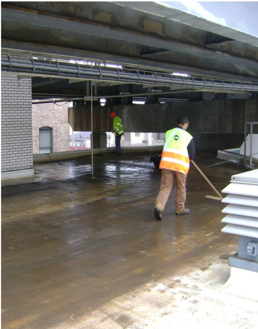
Pink Line California – Station roof
