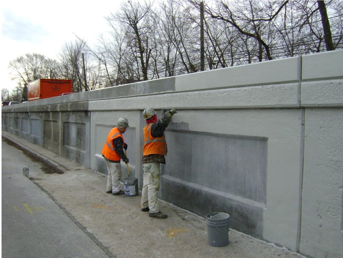
Applying Wall Sealer at Chicago Avenue Wall
