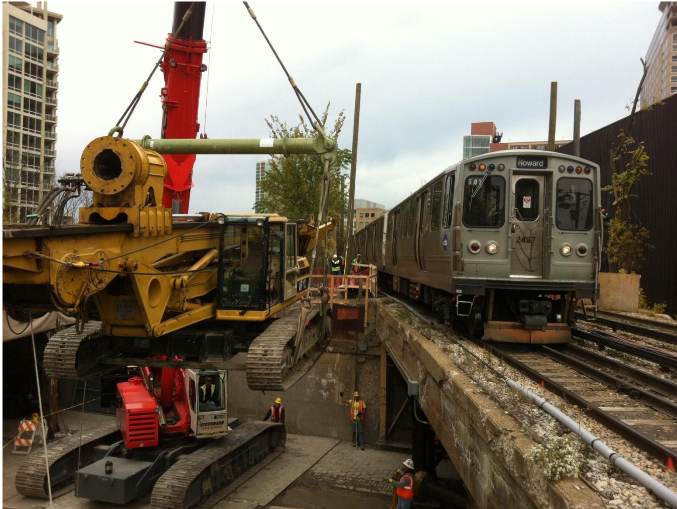
Lifting Drill Rig at Grove
