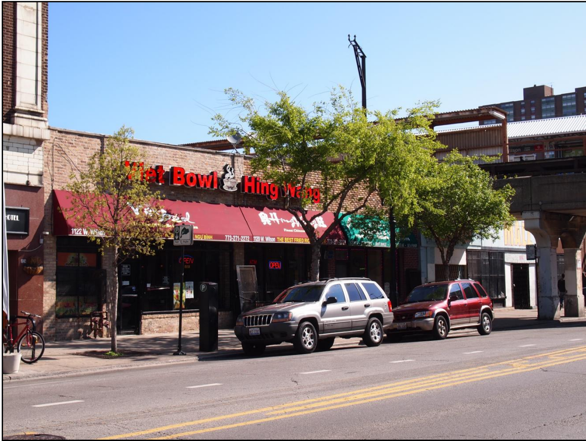
Plate 15. 1122 W. Wilson Avenue, view northeast.
