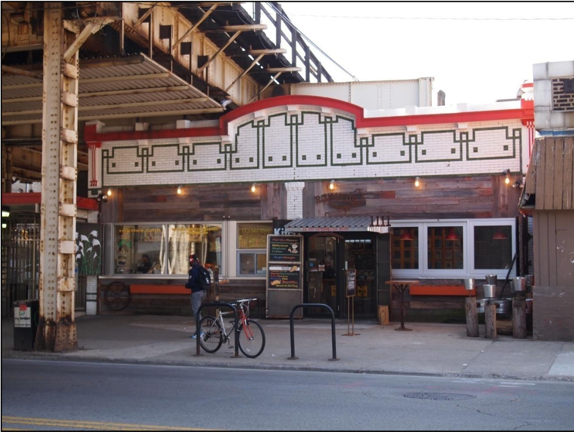
Plate 5. 1111 W. Wilson Avenue, proposed location of Wilson Main Station, view south.
