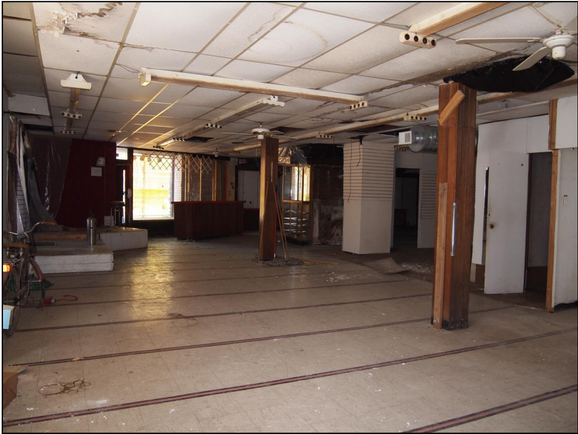
Plate 25. Interior of Majestic for Men store at 4620-4701 N. Broadway Avenue, view northwest.
