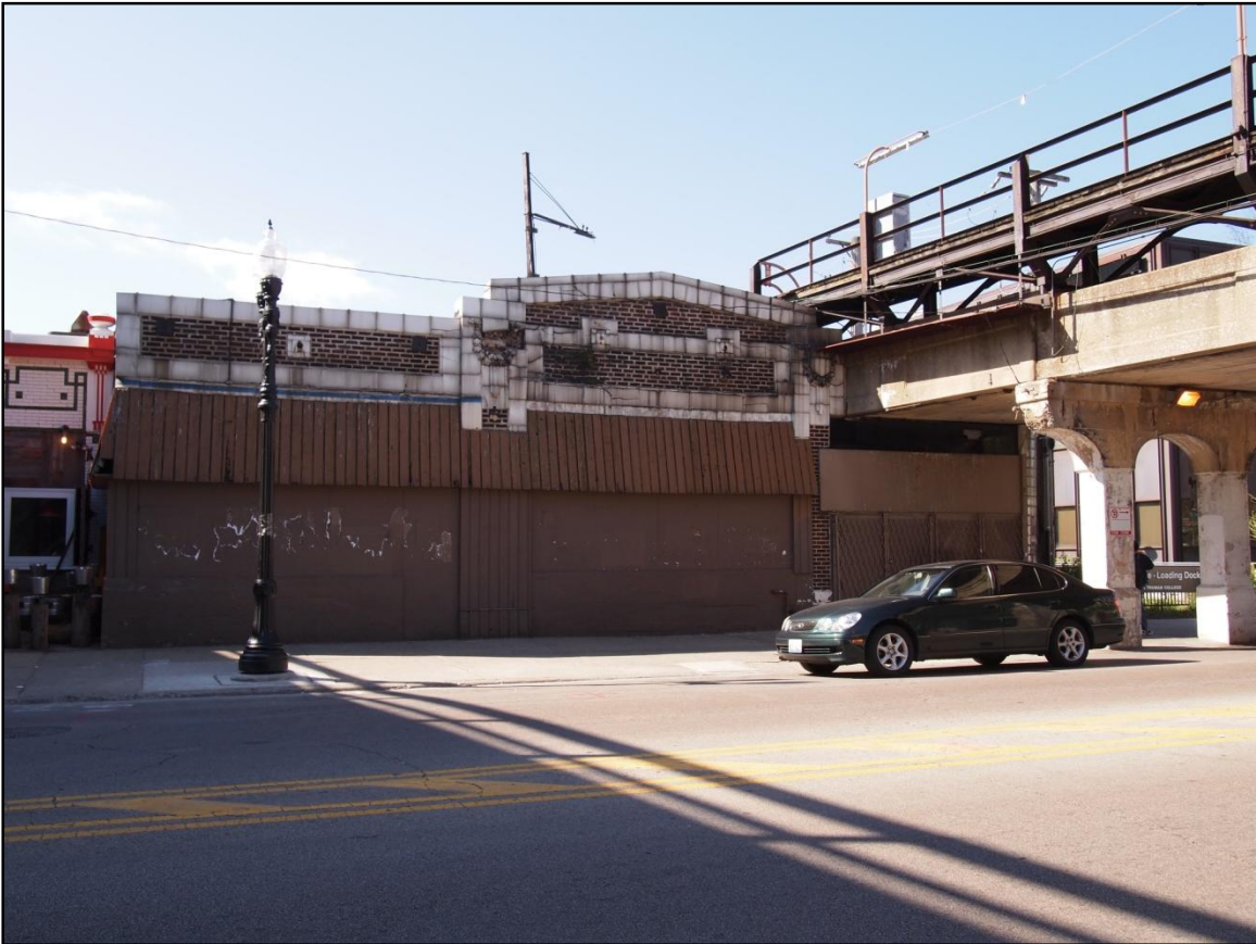
Plate 6. 1117 W. Wilson Avenue, proposed location of Wilson Main Station, view south.
