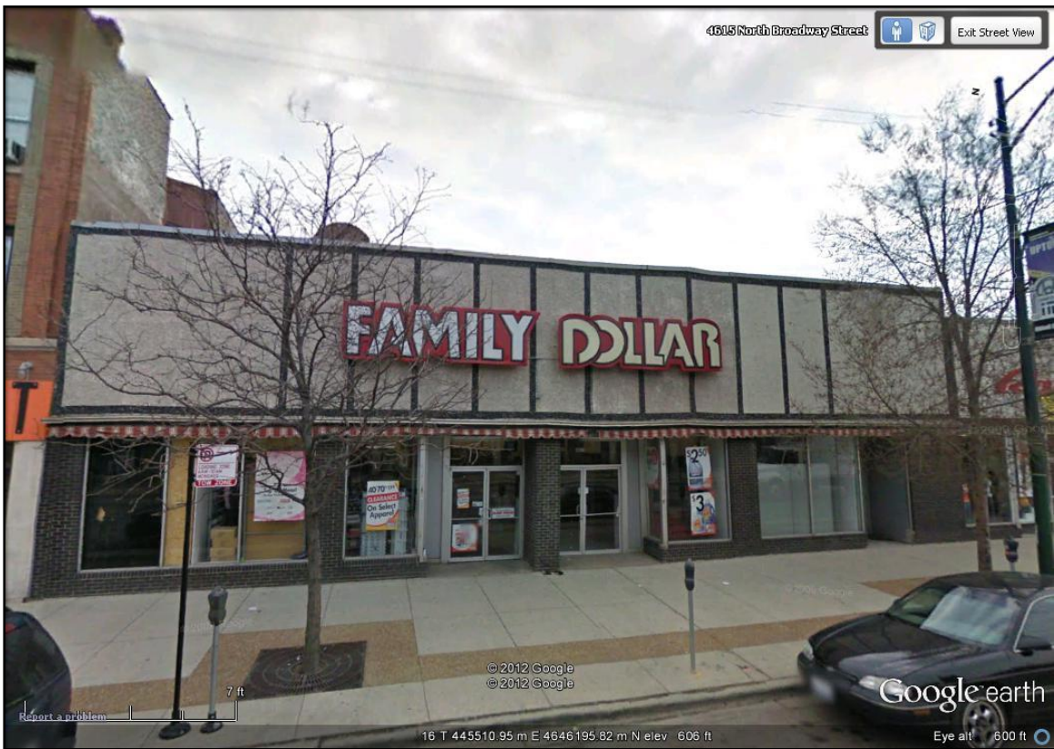
Plate 36. 4613-4617 N. Broadway Avenue, view east.
