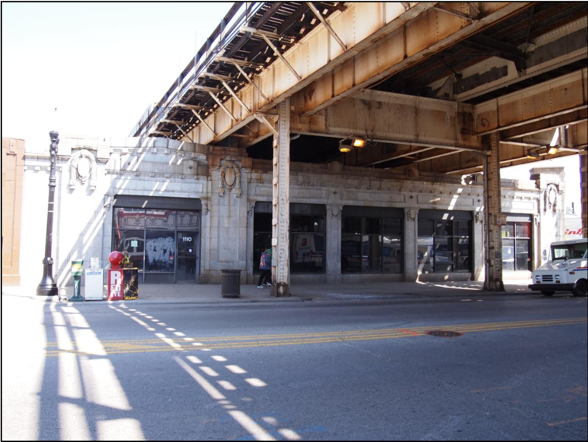
Plate 3. South elevation of Wilson Station, view north.
