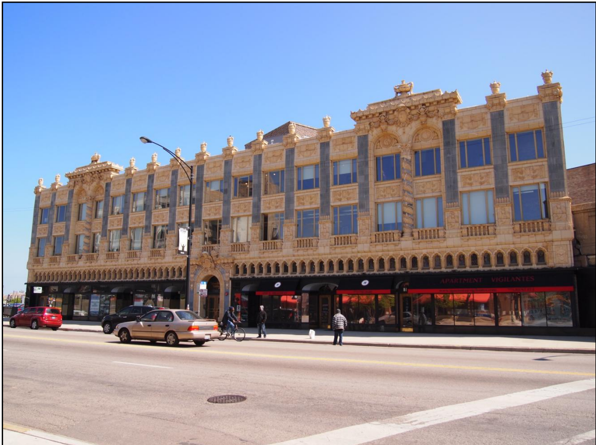
Plate 26. Uptown Broadway Building at 4701-4715 N. Broadway Avenue, view northeast.
