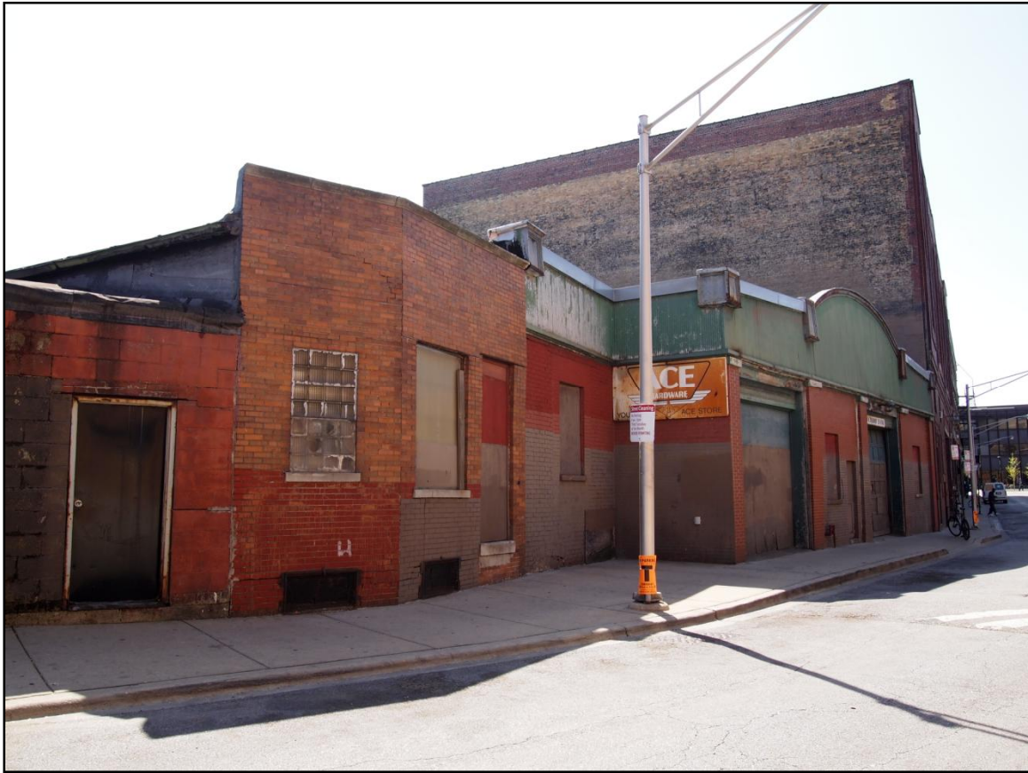
Plate 19. 4654 N. Broadway Avenue (fronts Clifton Avenue), view southeast.
