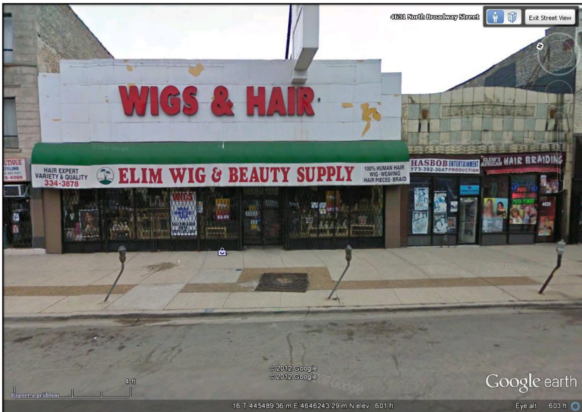
Plate 34. 4629 N. Broadway Avenue, view east.
