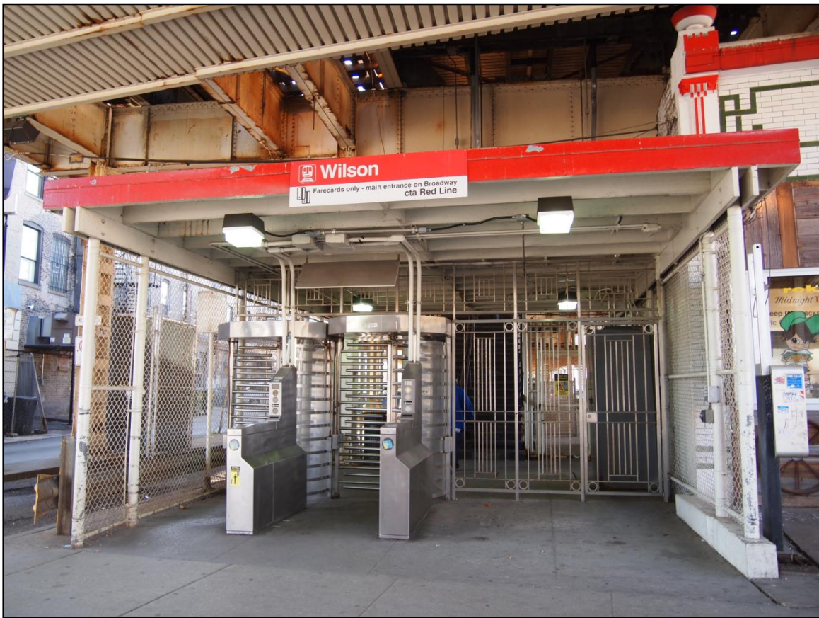
Plate 7. Existing Wilson Station auxiliary entrance, view south.
