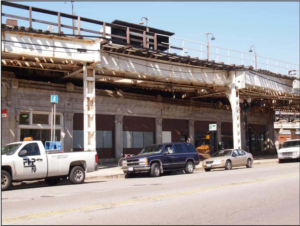
Plate 21. Wilson Station east elevation, view northwest.
