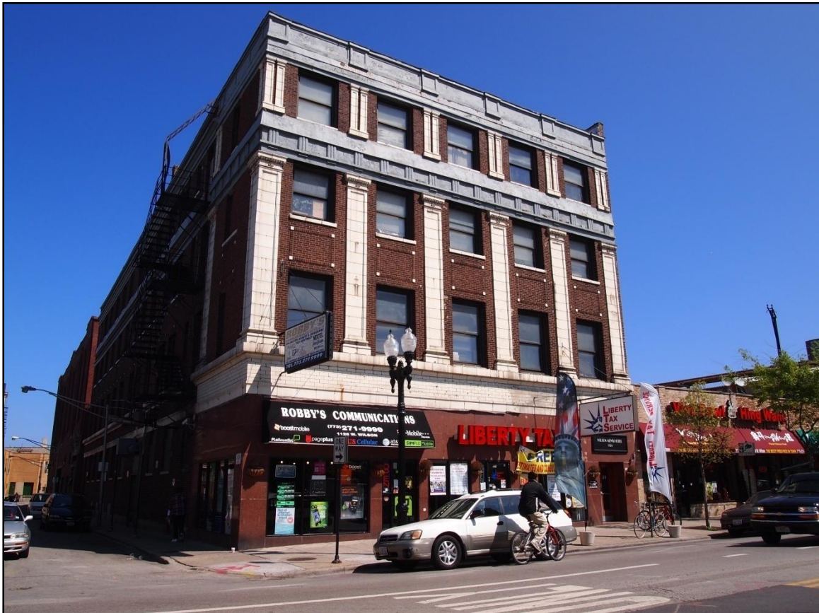
Plate 16. 1124 W. Wilson Avenue, view northeast.
