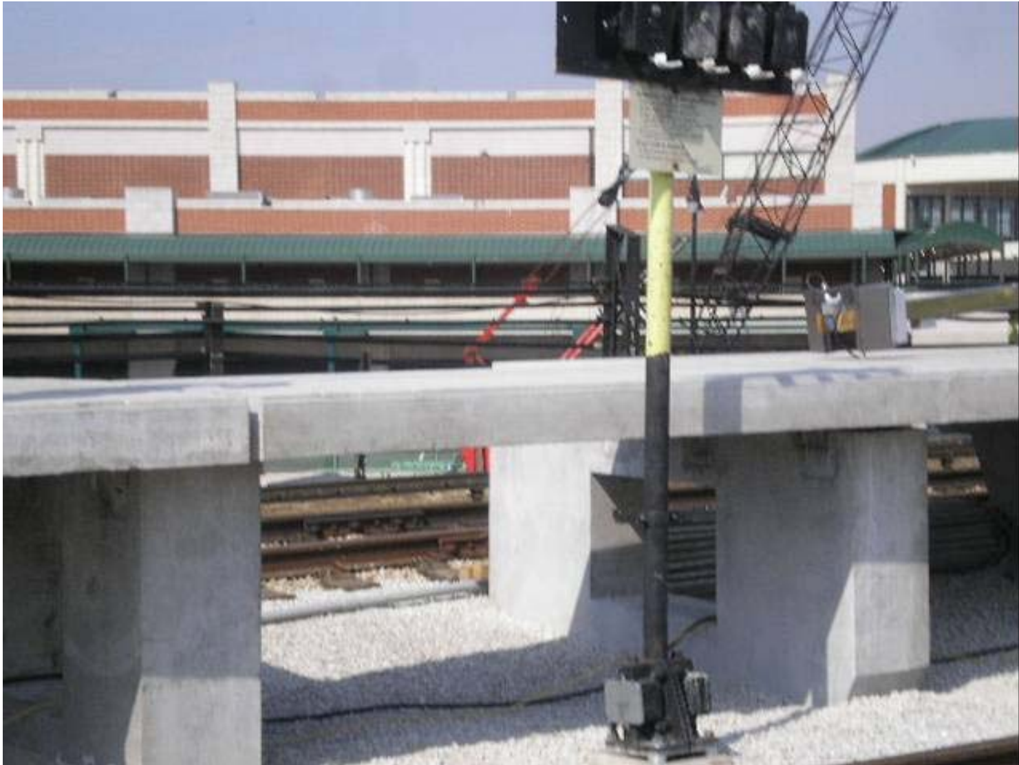
Side view of new concrete platform
