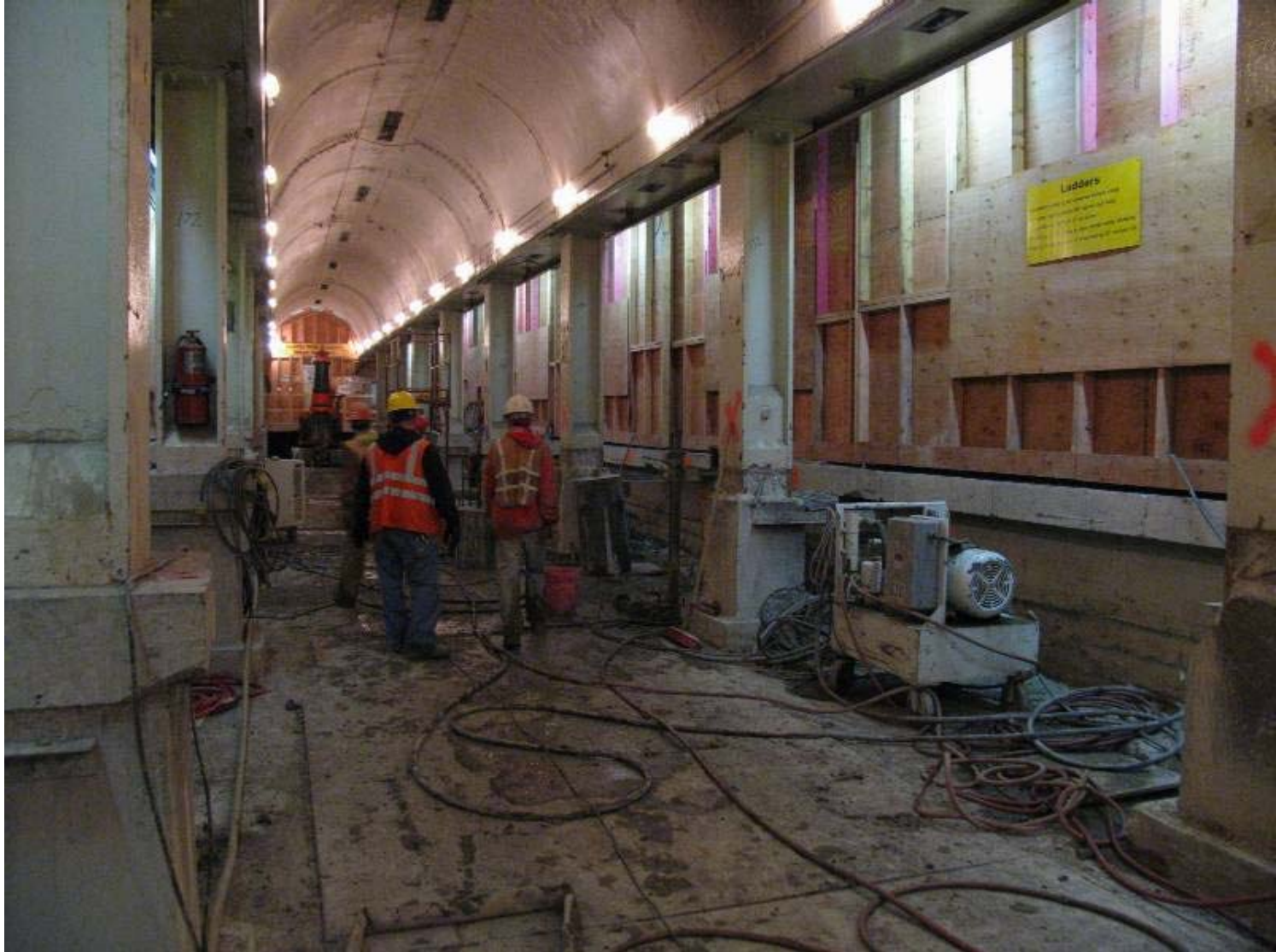
Washington Station (Red Line) subway platform removed for Block 37 track crossover
