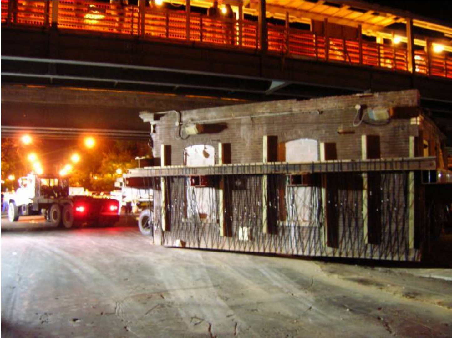
Fullerton historic station house move
