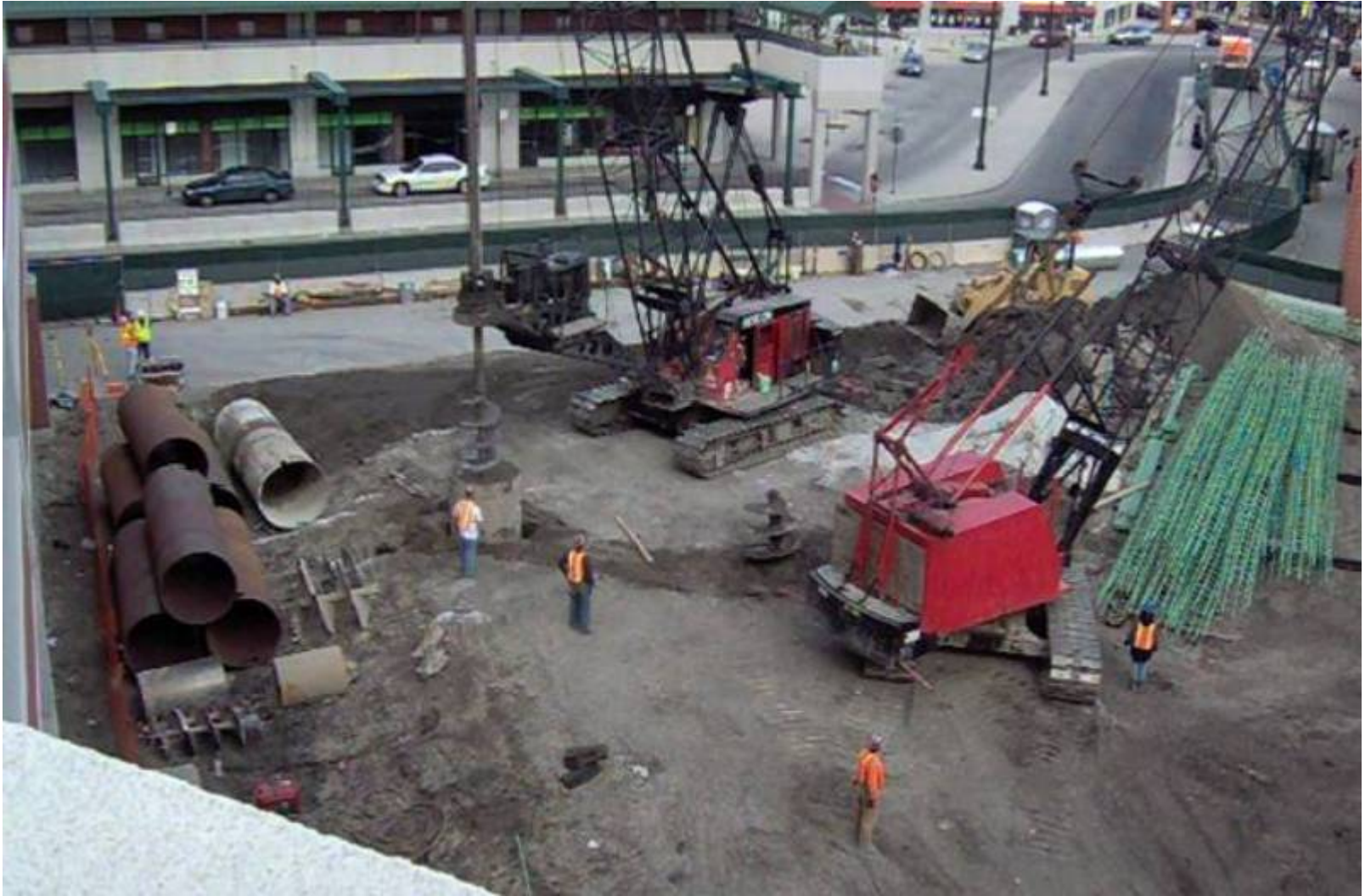
Caisson installation
