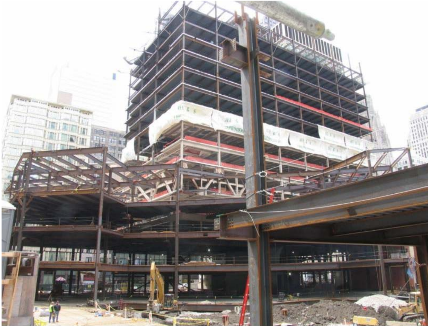
Block 37 retail office space
