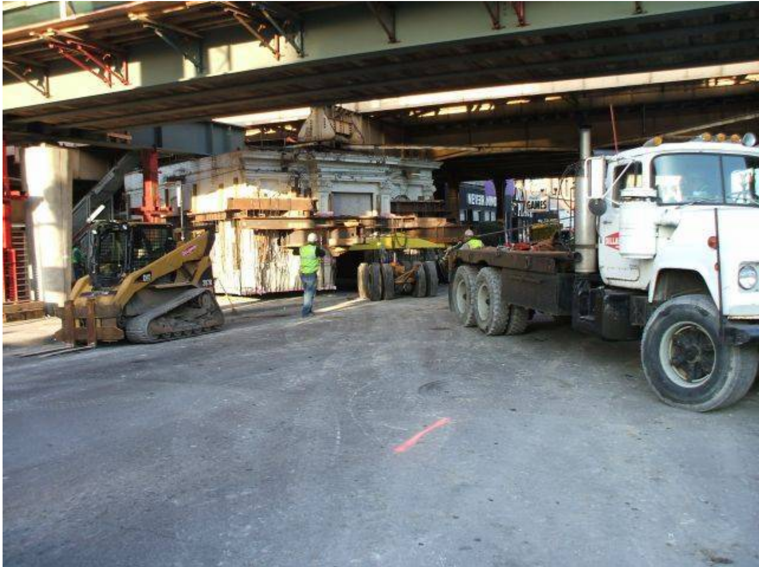
Belmont historic station house move (looking south)
