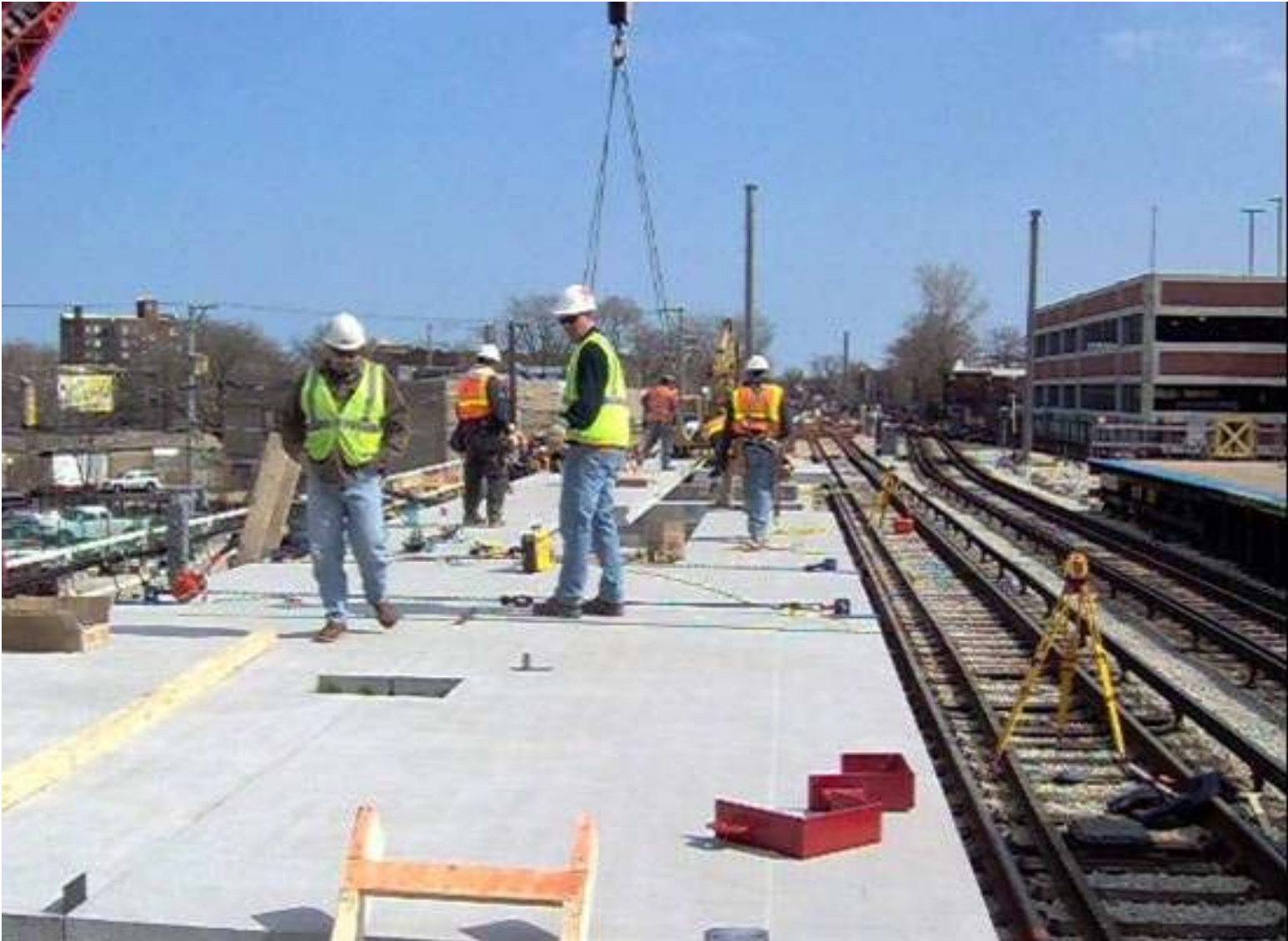
Concrete platform section at Howard Station
