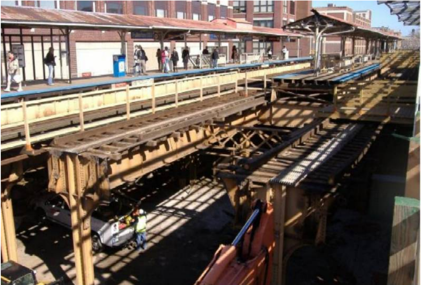
Fullerton Station old platform and old track 3 and 4 demolition
