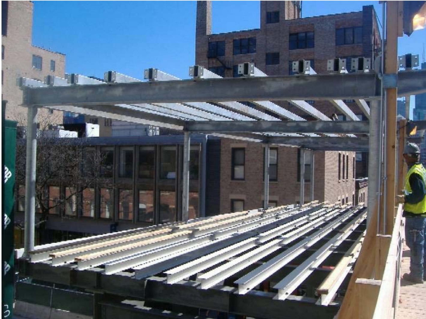
Steel work for new secondary entrance/exit at Chicago
