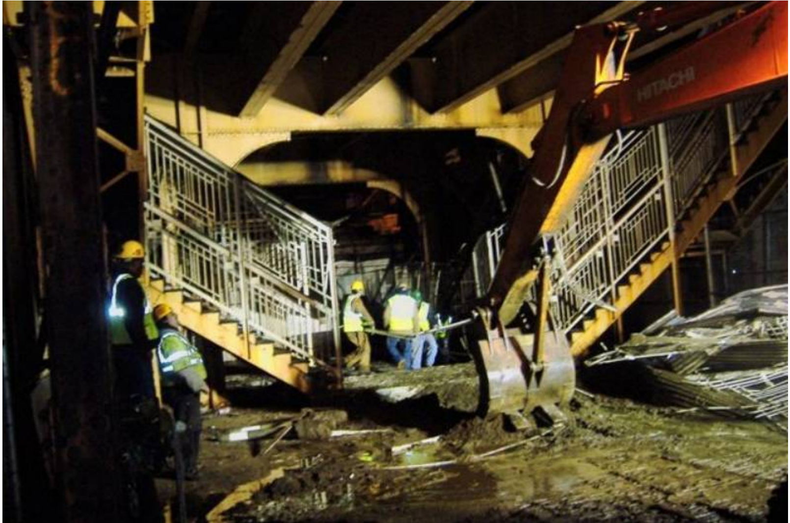
Demolition of Southport Station
