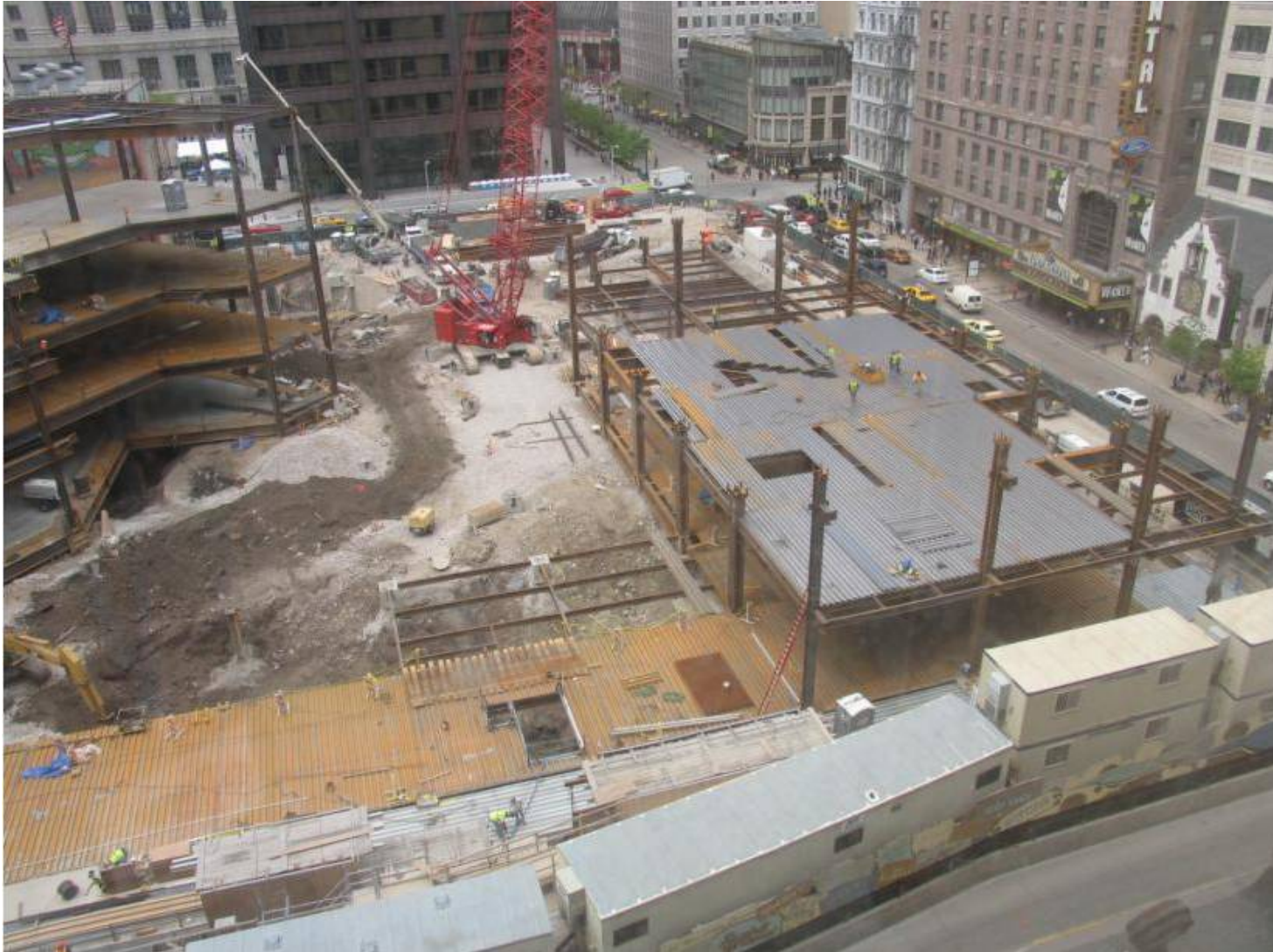
Block 37 work site
