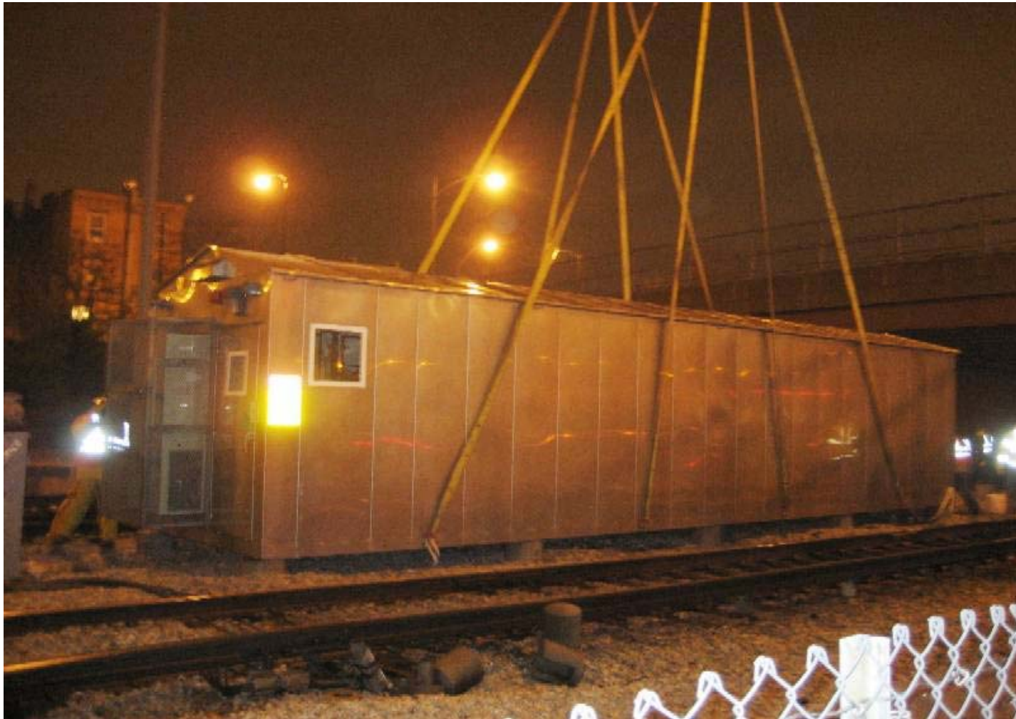
Installation of Pulaski relay house (Congress Line)
