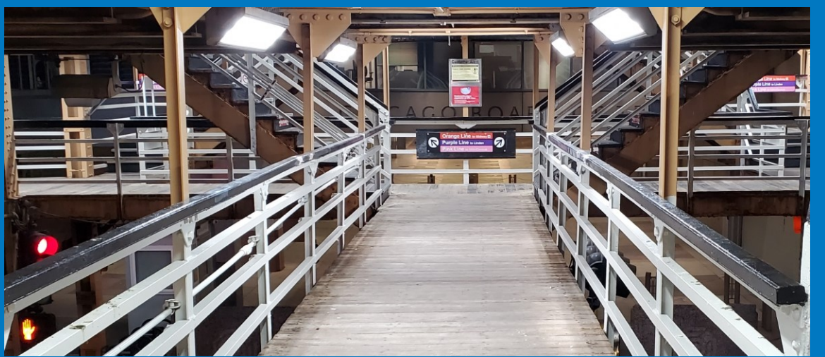
LaSalle/Van Buren mezzanine footbridge, before & after
